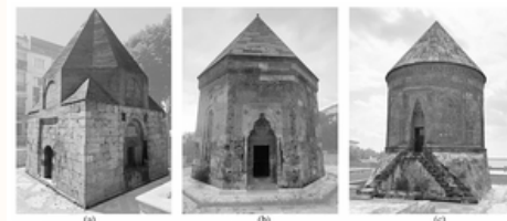
Fig. 2 Main body classes of kumbets. a Square, b polygonal, c circular. Image: authors
